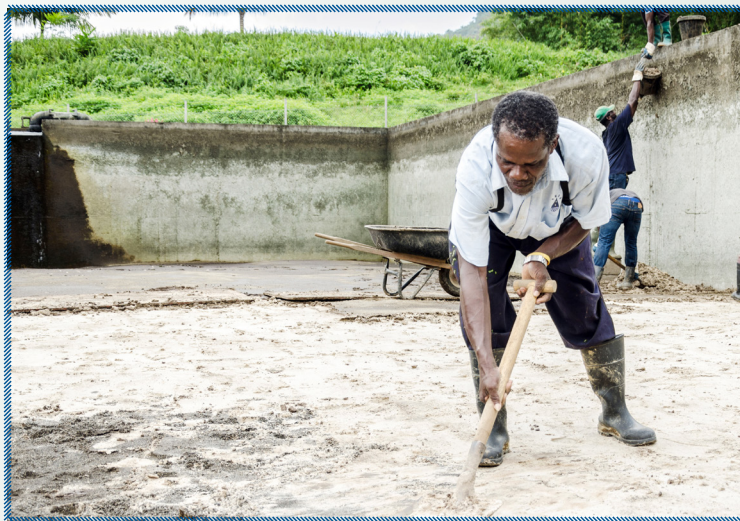
Resanding the filters at Dalaway
