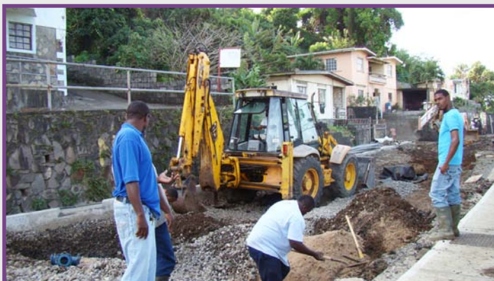
RUNNING PIPES AT THE FOUNTAIN STRETCH WHICH WAS BEING REFURBISHED AT THE TIME
