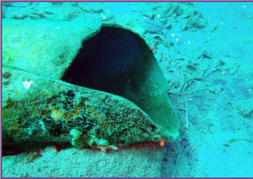
The damaged Sewer Outfall Pipe
